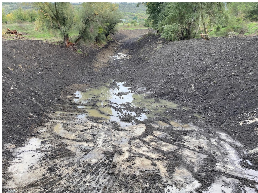
Figure 6. Improvement of the Botna riverbed upstream (approximately 500 m) of the mouth, autumn 2024
